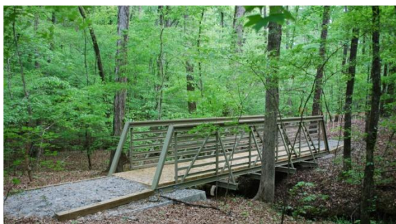
New trail bridge on the 1.5 mile relocation of the Buncombe Horse Trail
